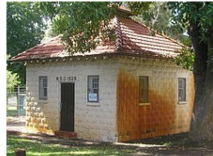
Iron III oxide staining caused by oxidation of dissolved iron(II) oxide and precipitation, from an unconfined aquifer in karst topography. Perth, Western Australia.
